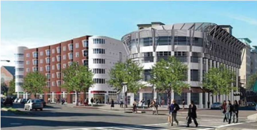
Fig. 1: Design and construction of the David Brower Center in Berkeley, CA, exemplified the missions of the environmental advocacy and nonprofit groups that will lease its office and meeting space
