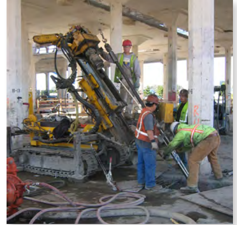
Figure 2: Battered micropile installation in an existing structure
