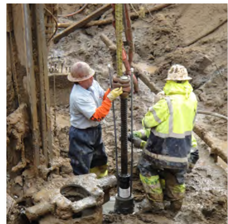
Figure 12: Installation of postgrouted micropiles
