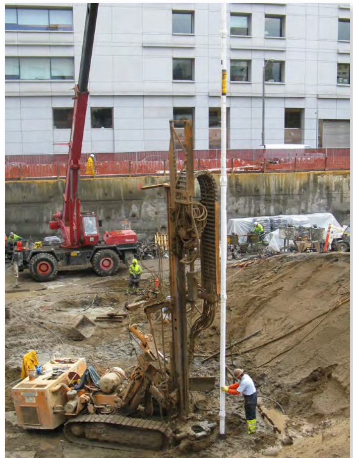
Figure 15: Micropile installation
