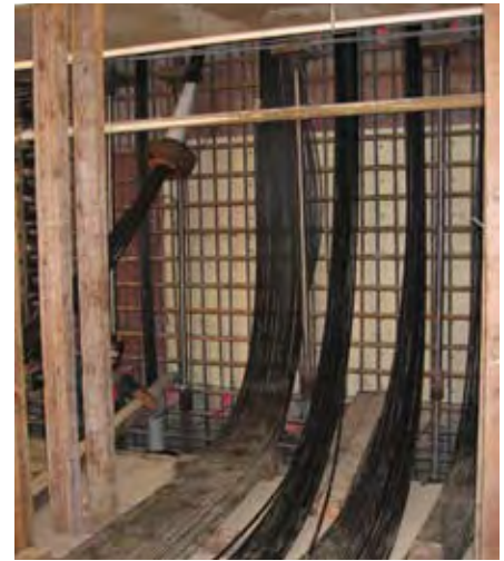
Fig. 6: Due to equipment constraints in the building, each strand for the bundled tendons was individually installed through the floor opening cut in the floor slabs
